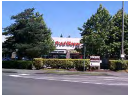
Building Mounted Signs Blocked by Trees
