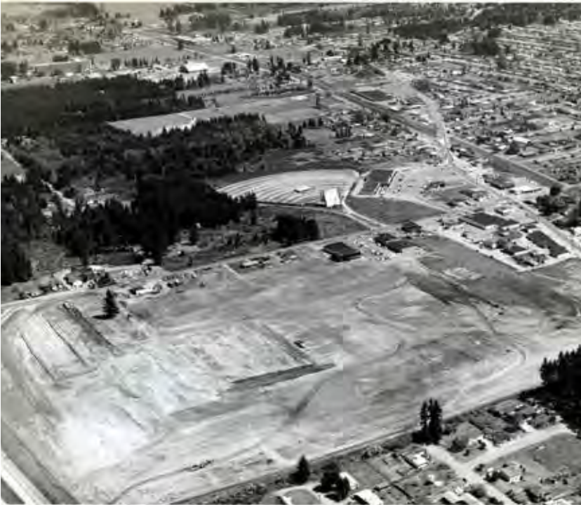
Figure 2. Sleater-Kinney Rd SE, South Sound Center Mall Construction, Drive-In Theater (1966)
