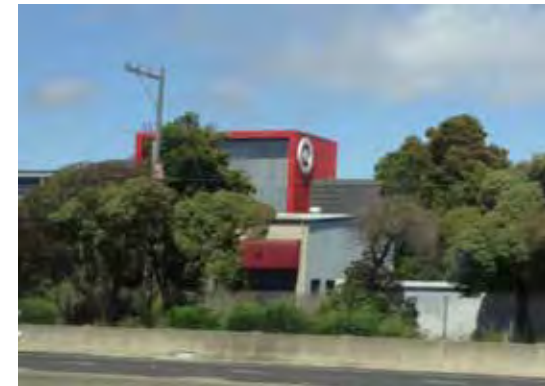
Visible Above Tree Line
