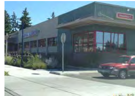
Retail Building Oriented to the Street
