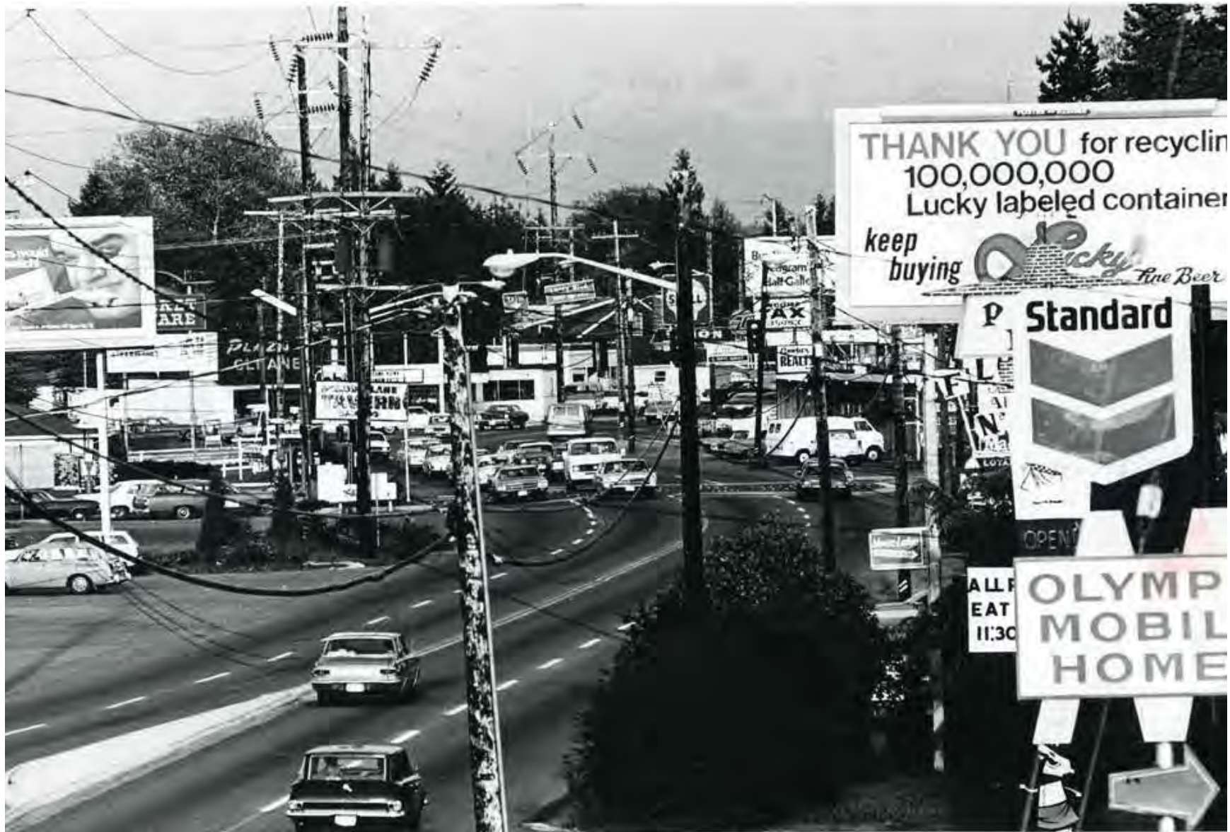
Figure 1. Pacific Avenue SE before reconstruction (1973)
