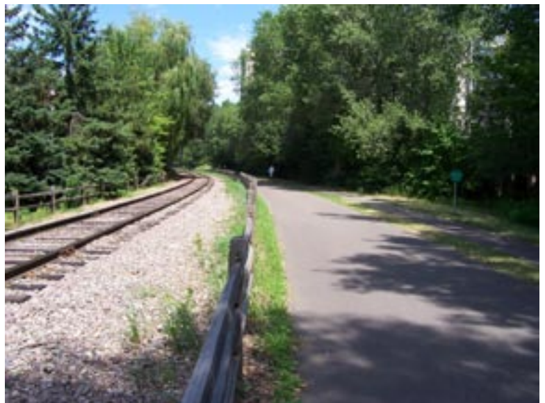
The Kennilworth Trail, an active rail with trail in Minneapolis, MN is separated from the railroad with a four foot fence. Photo by Paul Brewster.
