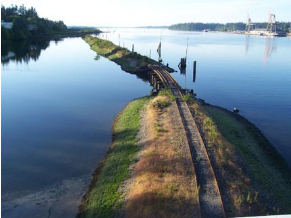
View of the future West Bay Trail Corridor as seen looking north from the 4th Avenue Bridge. The Port Lagoon to the left of the trestle provides winter habitat for waterbirds. Photo by Paul Brewster.
