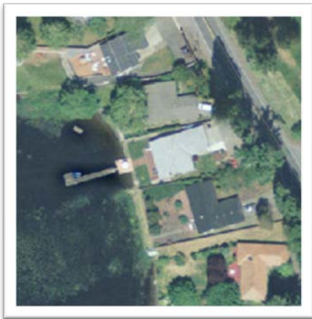
Homes in the center of the photo are less than 50 feet from the water's edge, and would be nonconforming under the proposed SMP update. Hicks Lake, Lacey.
