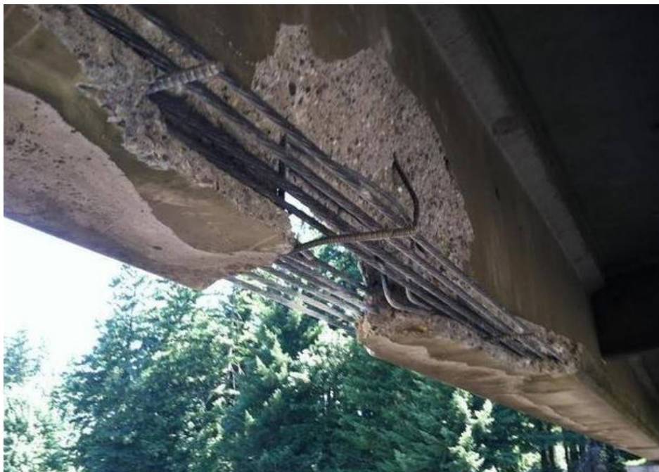
Figure 4-5: 93rd Avenue Bridge (2015)
