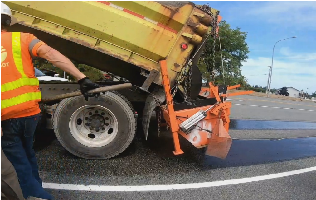
Figure 4-1: Wheel-path Chip Sealing
