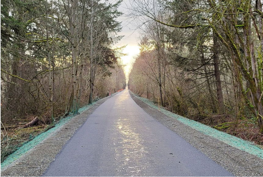
▲ Photo: Newly paved section of the Yelm Prairie Line Trail. [City of Yelm Image February 2024]
