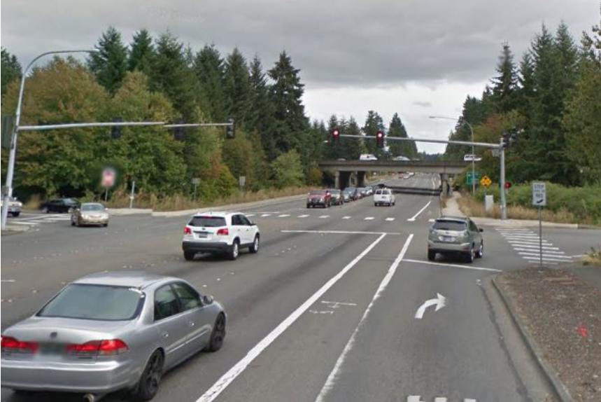
▲ Photo: Martin Way E looking eastbound at I-5. [Google Image September 2014]
