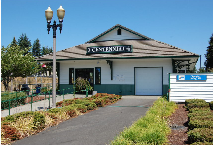
▲ Photo: Centennial Station, Olympia, WA. [WSDOT Image August 2009]
