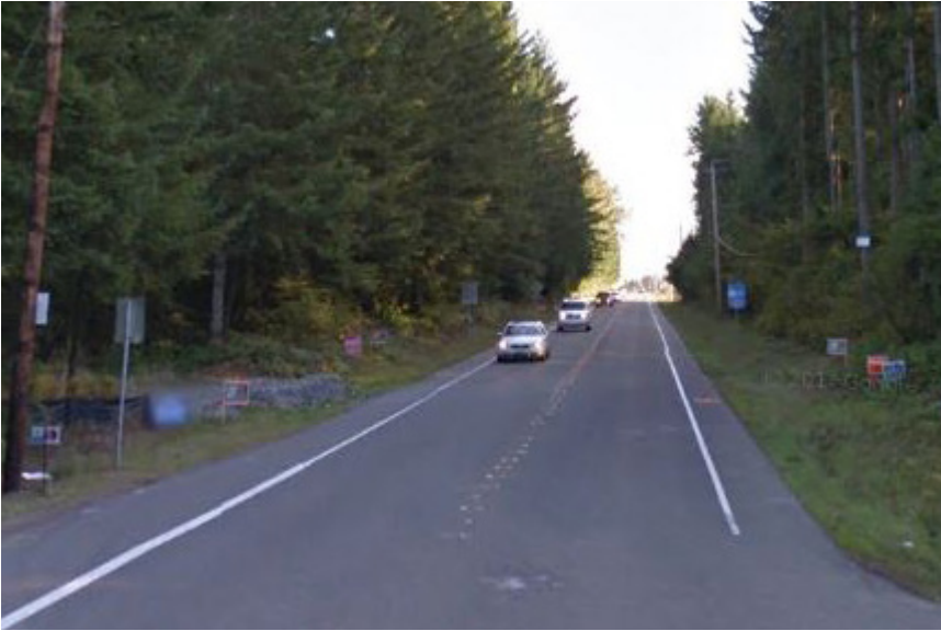
▲ Photo: Marvin Road NE looking southbound in the vicinity of 32nd Avenue NE. [Google Image October 2011]
