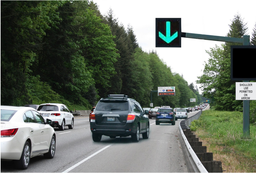
▲ Photo: An example of hard shoulder running on northbound I-405 near Lynnwood. [Washington State Department of Transportation Image]
