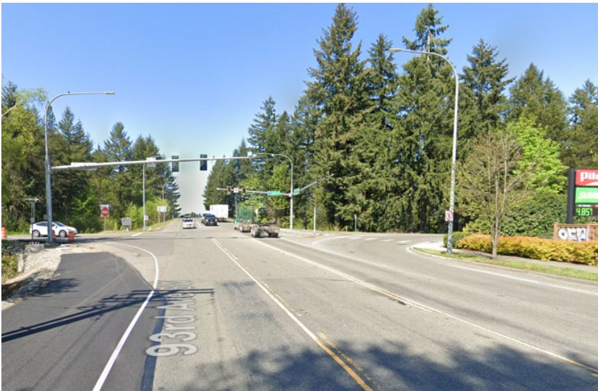
▲ Photo: 93rd Avenue Southeast looking westbound at the northbound ramps of I-5. [Google Image May 2023]
