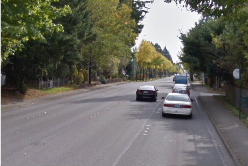
▲ Photo: College Street SE looking southbound in the vicinity of 31st Avenue SE. [Google Image October 2011]
