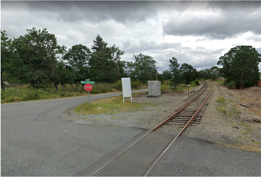
▲ Photo: BNSF railroad looking east near the intersection of Union Mills Road SE and Mayes Road SE. The extension of the Karen Fraser Woodland Trail would utilize this existing railroad line. [Google Image June 2019]
