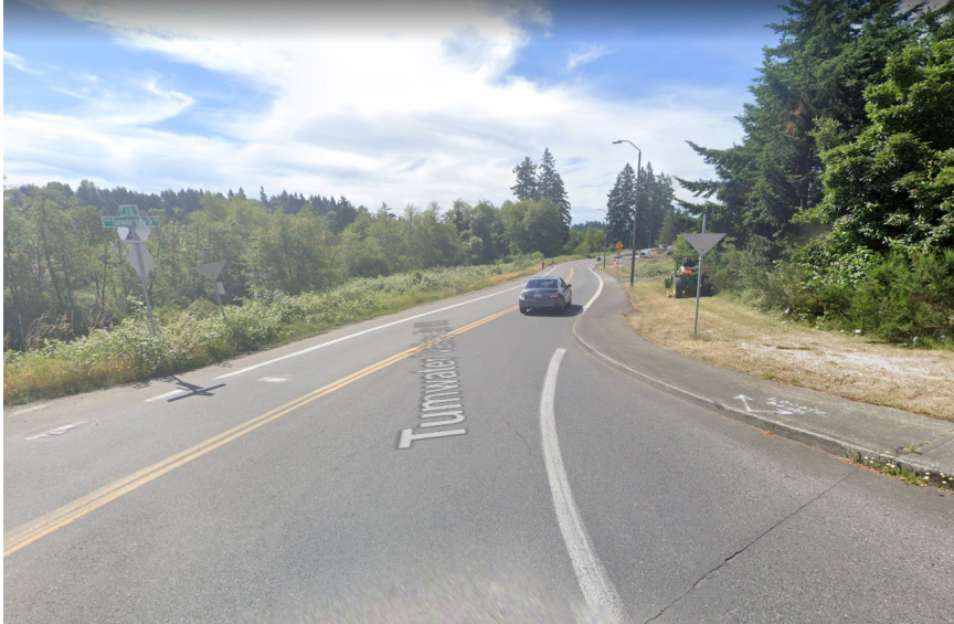
▲ Photo: Tumwater Valley Drive SE looking southbound, just south of the intersection with E Street. [Google Image June 2019]
