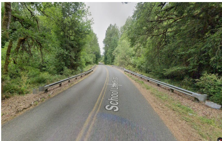
The S2 Bridge on School Land Road.
