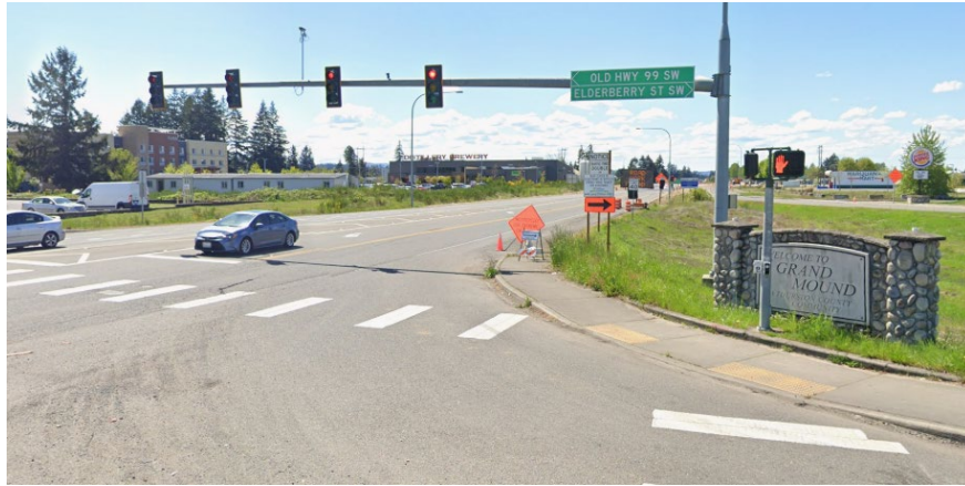
The intersection of Elderberry St SW and US 12 is signalized with marked pedestrian crossings.
