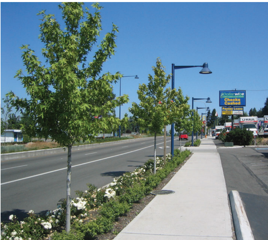
Street improvements on Pacific Highway
