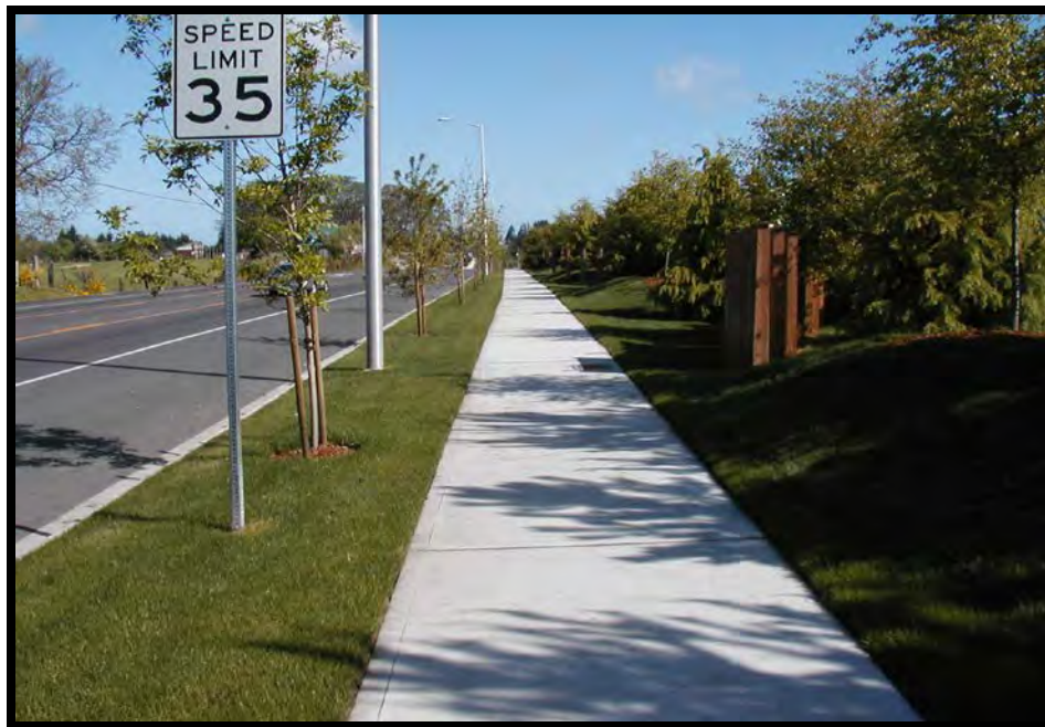
Photo E. View of a well-designed planter strip, however tree wells are not adequate – turf is too close to tree's rootball.
