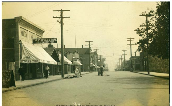
Historic structures in downtown Tenino often included unique detailing.
