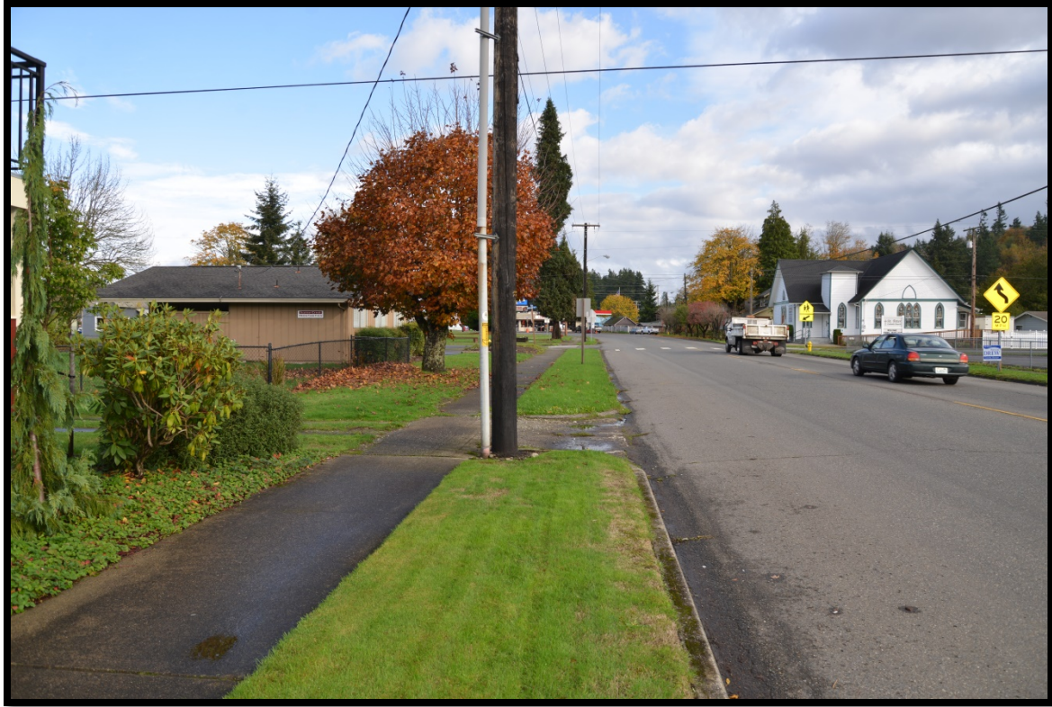
Photo C. Planter strips under power lines. Space is there for utility friendly trees.
