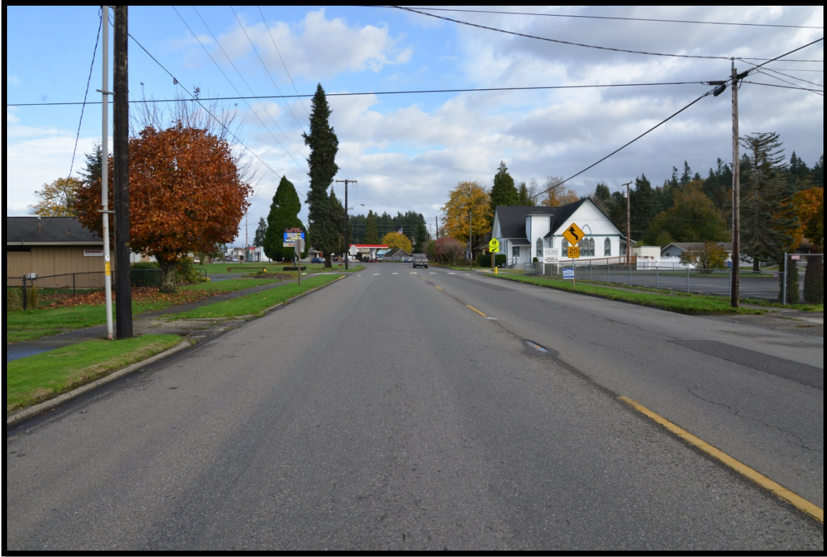
Photo G. Plenty of space for trees, with some overhead powerline restrictions.
