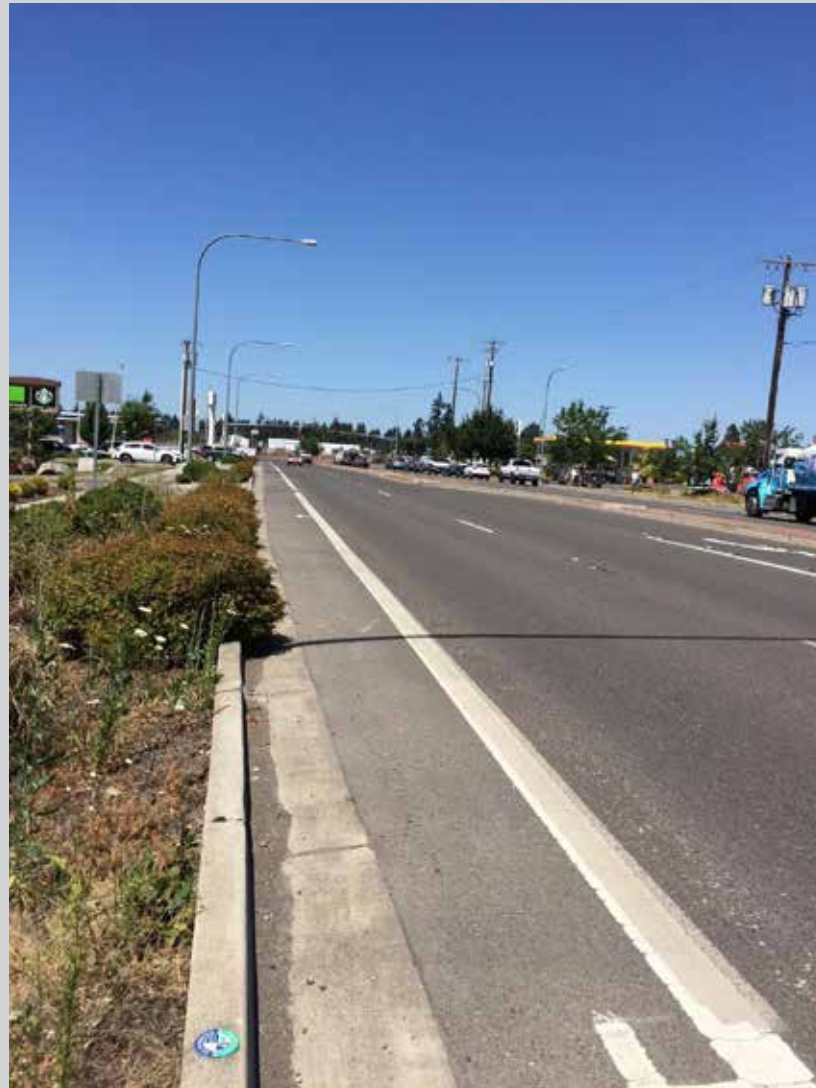
FIG 29: Old Highway 99's paved shoulder is separated from the adjacent travel lane by a solid stripe and provides a key north-south route for cyclists in Grand Mound.
