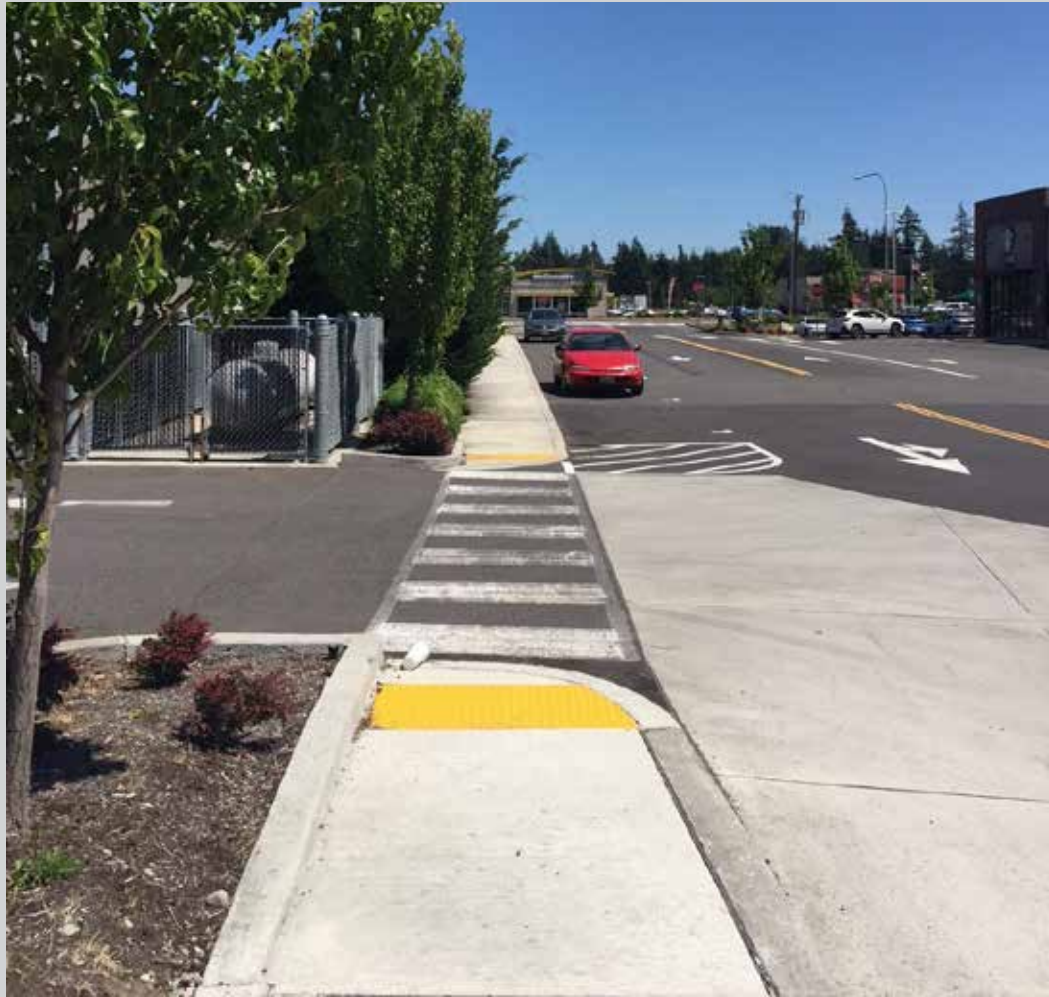
FIG 27: Sidewalks, curb cuts and marked crossings support safe walking between a new hotel, restaurants and other commercial businesses near the intersection of Old Highway 99 and US 12.
