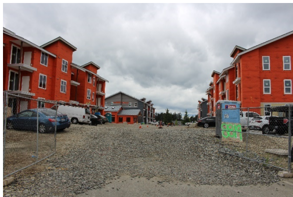
New market-rate apartments under construction.
