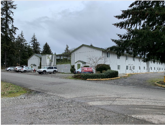
Older apartment building.
