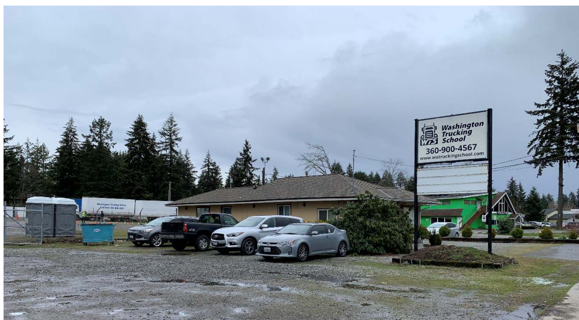
Figure 20. Much of the Martin Way Corridor is developed at relatively low intensities, such as this property in the Carpenter to Marvin segment, which has a small, single-story building and a large open area dedicated to parking.
