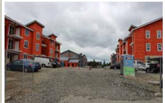
New market-rate apartments under construction.
