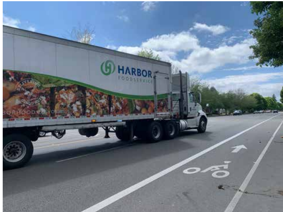
Figure 25. Bicycle lanes on Martin Way are immediately adjacent to travel lanes with heavy traffic volumes.
