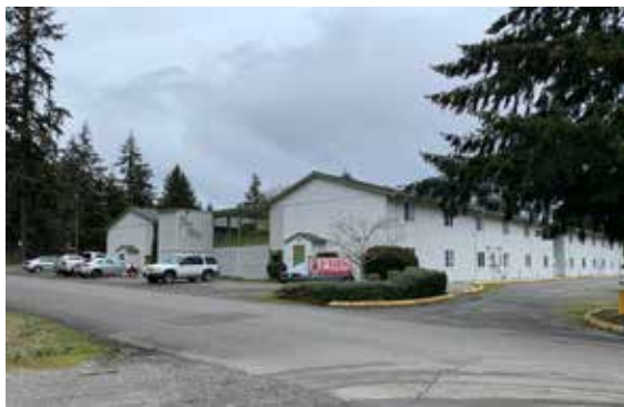
Older apartment building.
