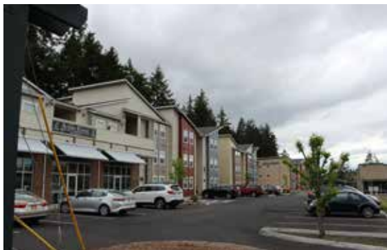
New mixed-use professional offices and apartments.
