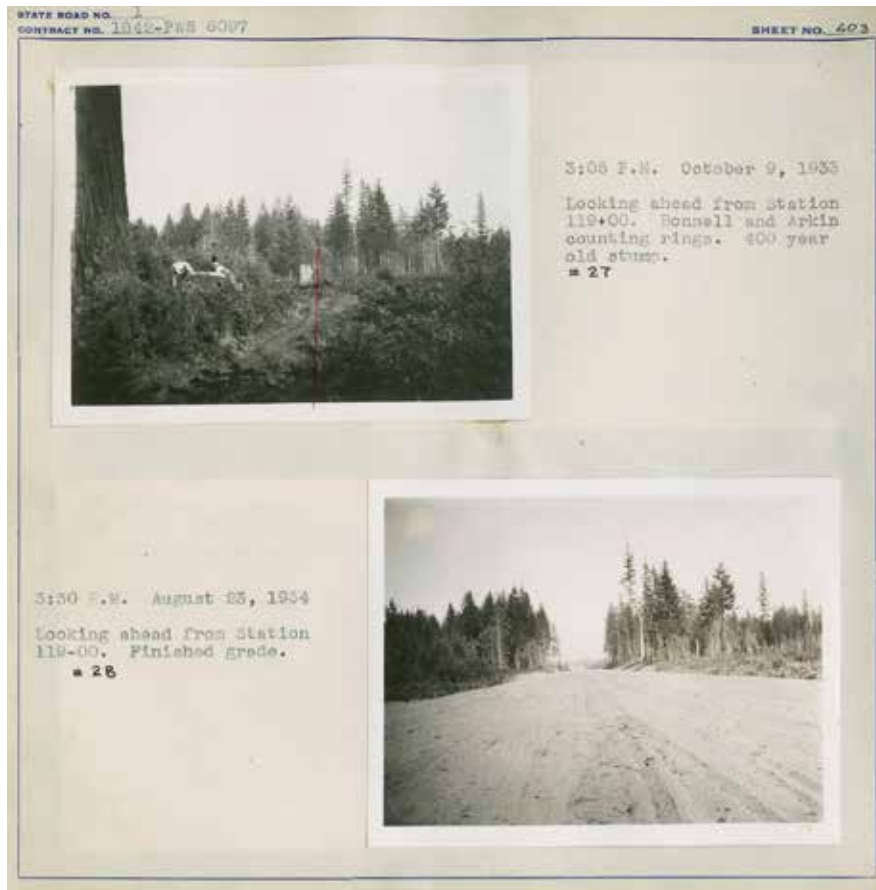
Figure 3. Survey records show the thickly forested terrain that was cleared and graded to build Martin Way. The top photo was taken in 1933, before road construction, and includes a 400-year-old stump. The bottom photo shows the same location in 1934. Source: Washington State Archives
